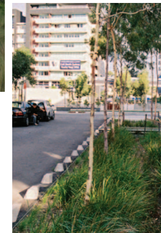
Flush kerb and swale
